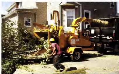
Figure 6. Regulated materials chipped to less than 1 inch in two dimensions can move out of the regulated area.
